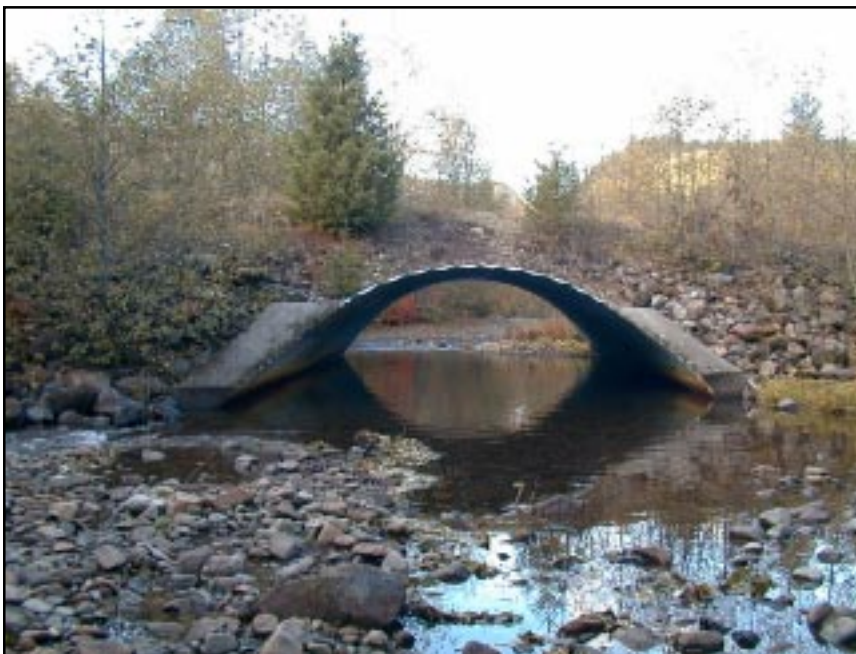
Photo 2.3 A bottomless arch pipe culvert that spans the active stream channel and doesn't constrict the flow, maintains a natural stream bottom, and helps promote fish passage. (Photo provided by S. Wilson-Musser)
