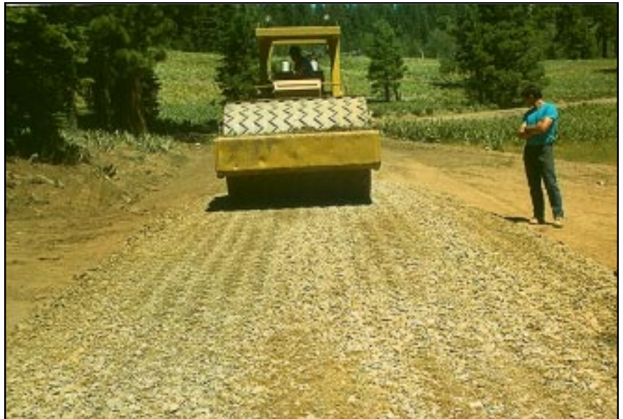
Photo 12.4 A grid roller can be used to produce a desirable surfacing material when the coarse rock is relatively soft. Level and compact the roadway surface aggregate to achieve a dense, smooth, well-drained riding surface.
