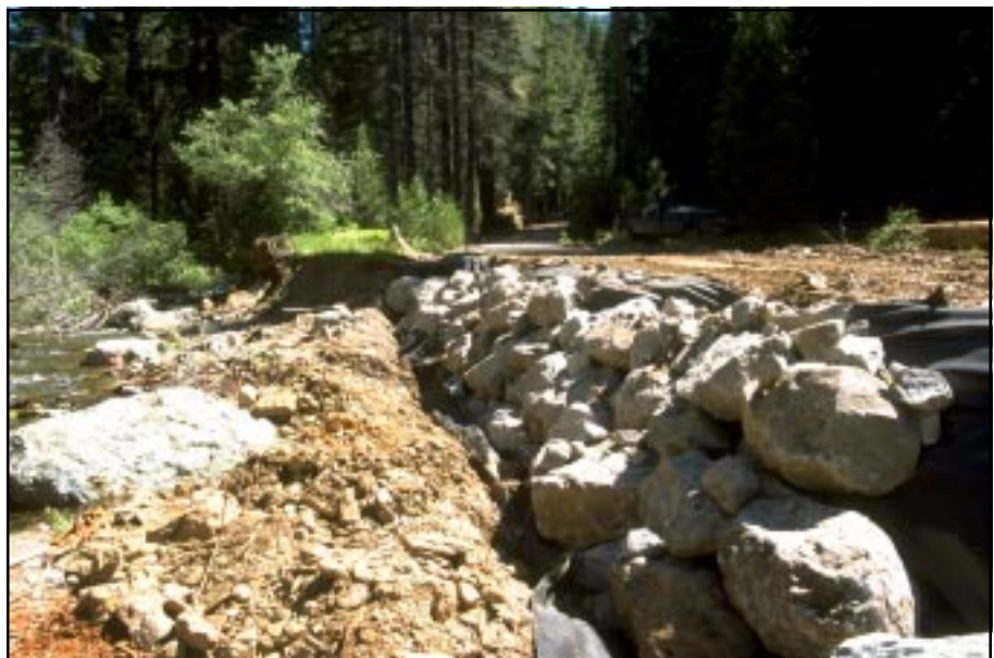
Photo 6.7 Riprap with a geotextile filter backing are being used to protect the road from high water flows. Note that the road is poorly located so close to the stream!
