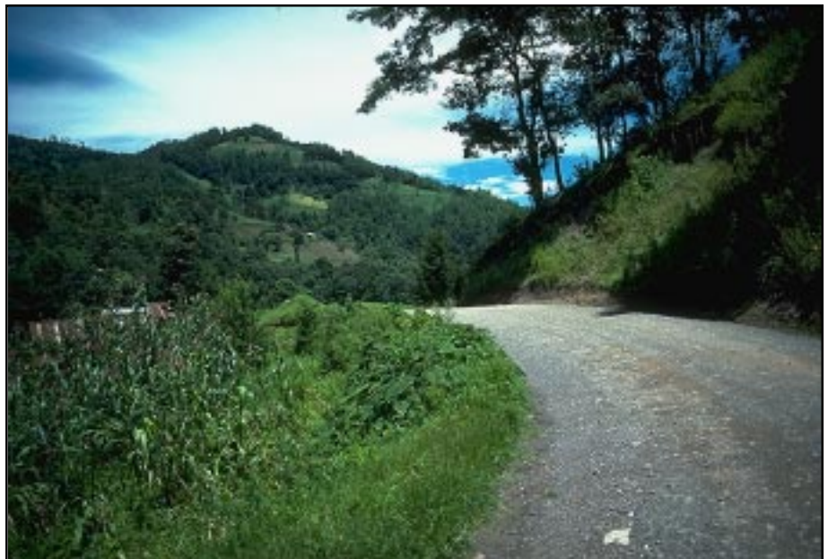
Photo 2.5 A well designed, “minimum impact” road that has an appropriate standard for its use, good drainage, and stable slopes.
