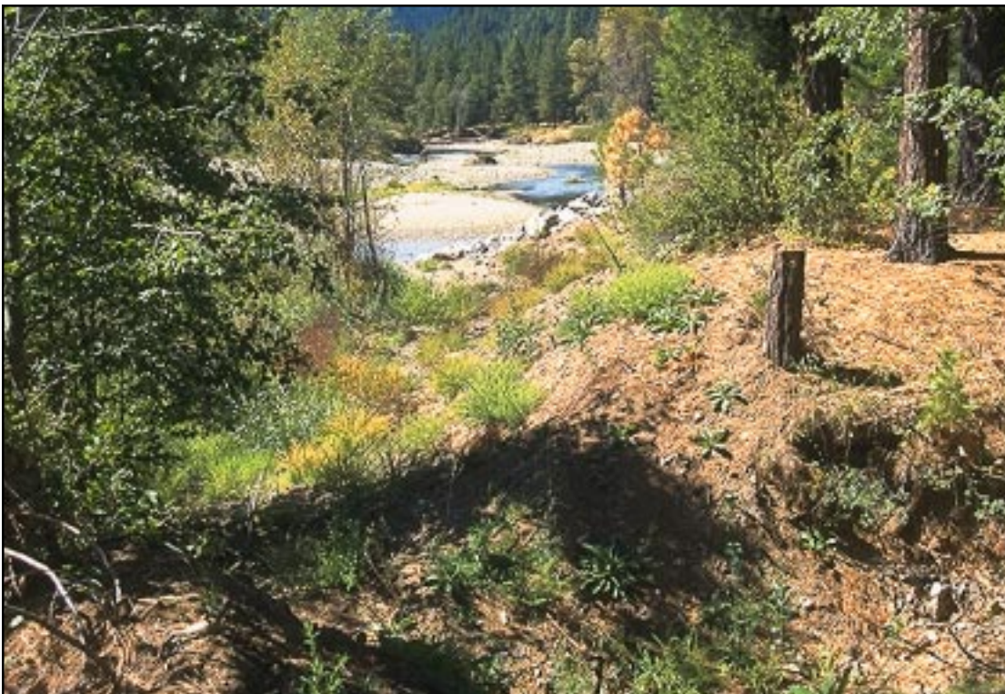
Photo 4.12 Close roads that are not needed. Stabilize the surface with water bars, berms, and ground cover such as grass seed and mulch.
