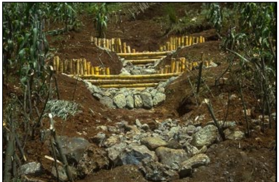
Photo 14.4 Construct debris retention and gully control structures with a notched wier to keep flow over the middle of the structure, add scour protection at the outlet of each structure, and key the structures into the firm soil banks.
