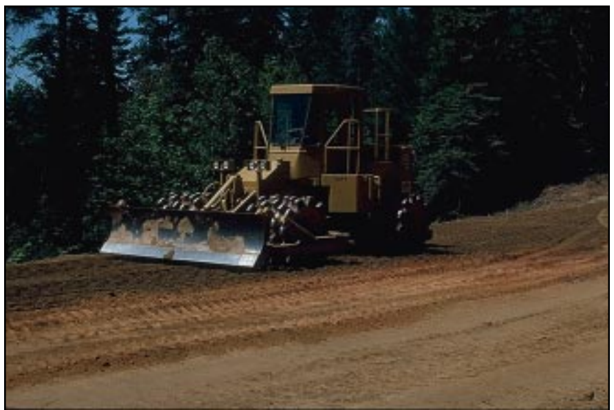
Photo 12.5 Compaction of soil and aggregate is typically the least expensive way to improve the strength and performance of the material. Compaction is useful and cost-effective both for the stability of fill embankments and for the road surface.
