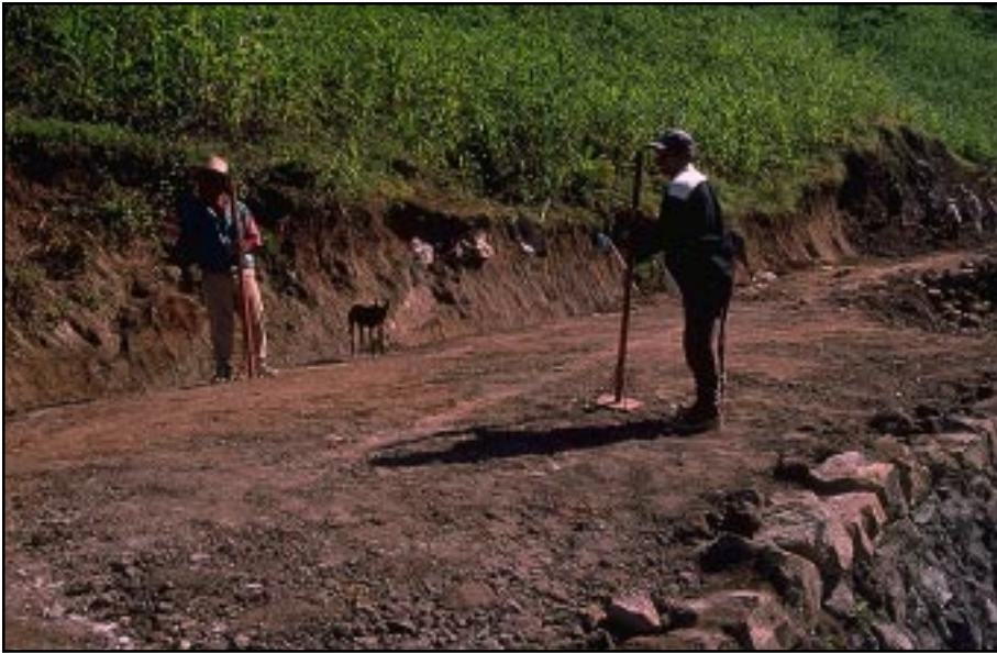
Photo 11.6 Simple hand compaction behind a low rock wall. Compaction is important behind any retaining structure or fill. It can be achieved by hand or, preferably, using equipment such as a wacker or small compactor.
