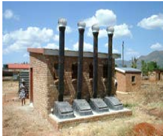
An "enviroloo" (dry composting toilets) mandated by the Department of Public Works in the Northern Province of the Republic of South Africa (2002)
