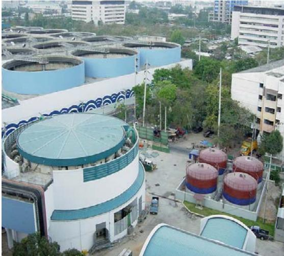
Managed by the Bangkok Metropolitan Administration in Bangkok city, the Dindaeng Water Environment Control Plant operates a combined wastewater collection and treatment system with screening and grit removal, biological activated sludge with nutrient removal, and final clarification.
