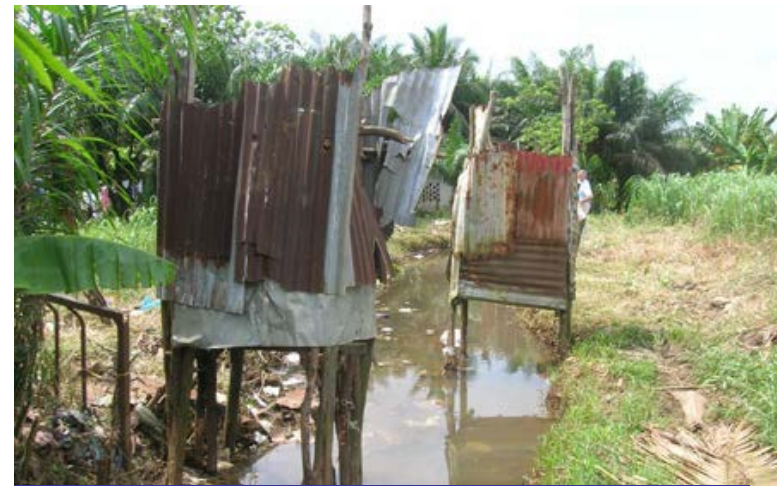
Total failure of latrines to contain pathogens
