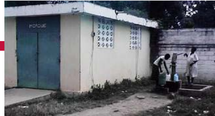
Potable water supply near hospital morgue
